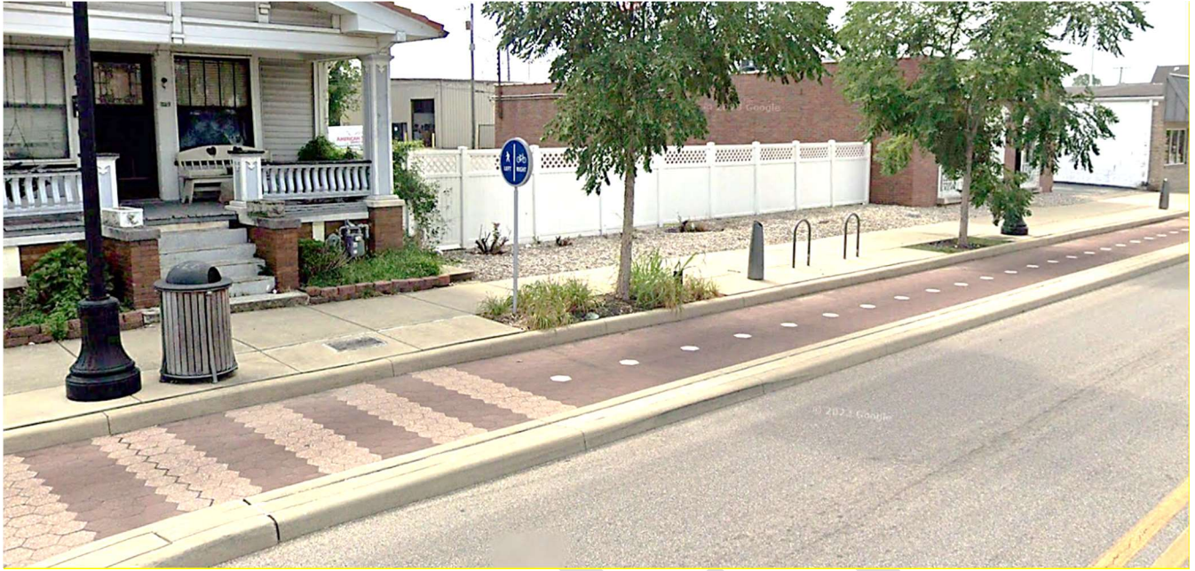
FIGURE 11 - EVANSVILLE, INDIANA EXAMPLE OF A COMPLETE STREET, SEPARATED BIKE LANE (ITSELF WITH SIGNAGE AND CLEAR DIRECTIONAL CUES), BIKE RACK, AND WIDE SIDEWALK WITH GREENERY AND A WASTE RECEPTACLE. SOURCE: GOOGLE 2023.
